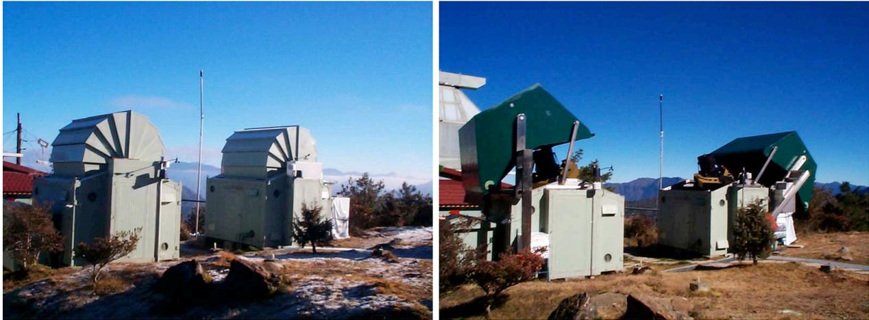
Figure 3. Left panel: TAOS I enclosures with original lids. Right panel: same enclosures with new lids.
