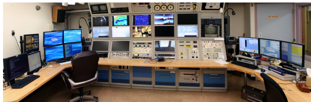
Figure 6 (a) Summit control room
